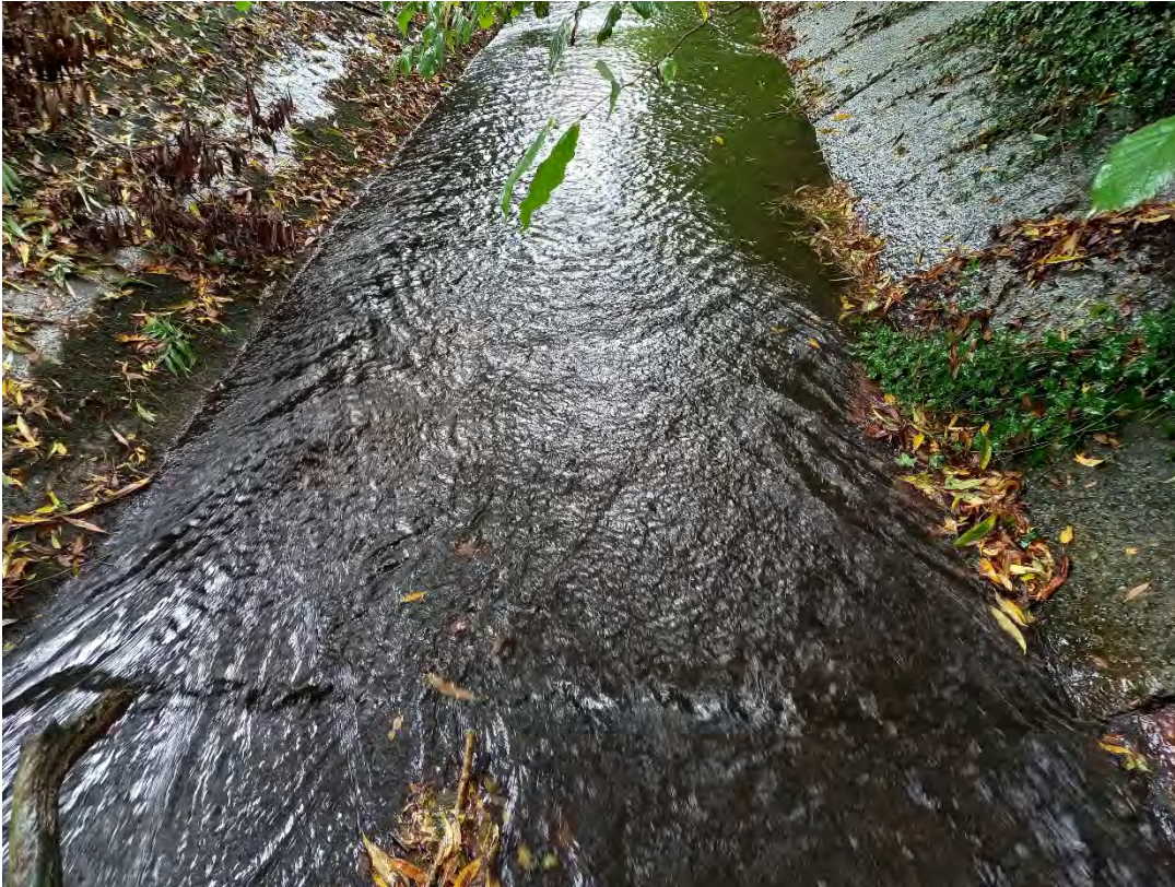
Figure C-18 Site 34 US Impacted
