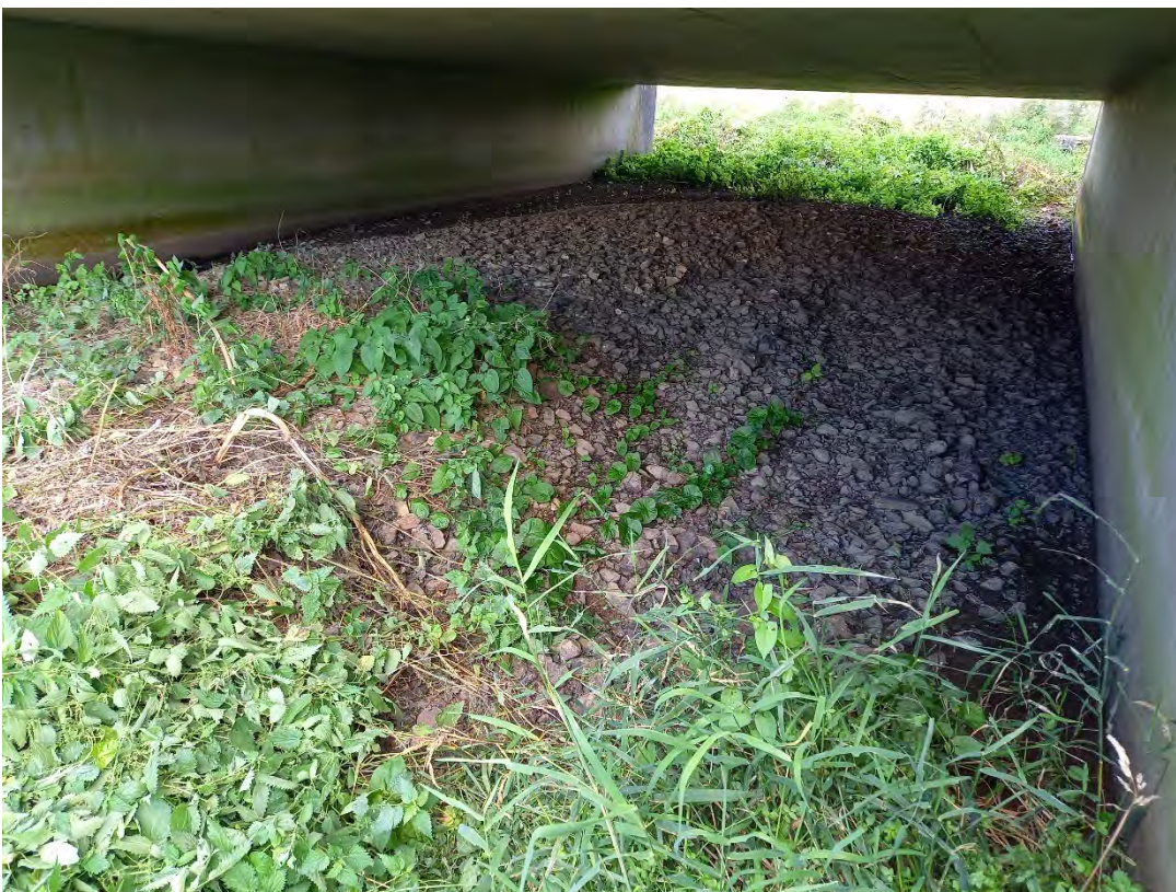
Figure C-29 Site 52 DS Impact
