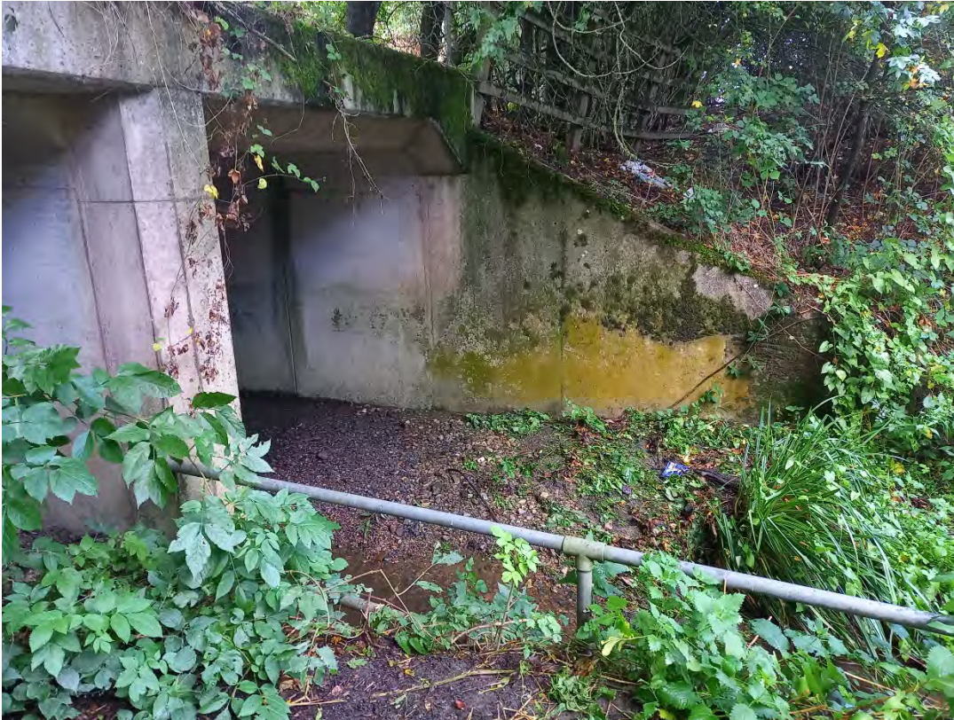
Figure C-20 Site 36 DS Impacted
