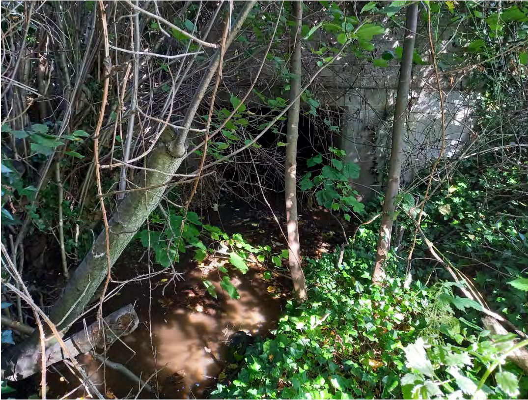
Figure C-11 Site 24 DS Impacted
