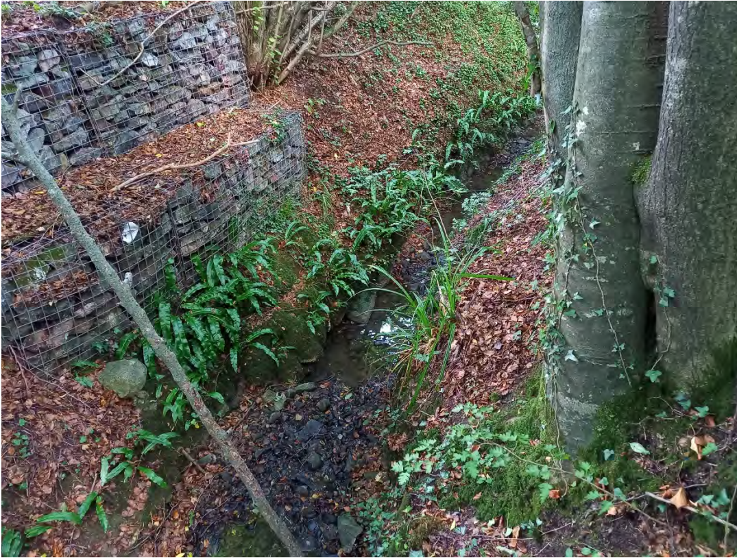
Figure C-15 Site 31 DS Impacted
